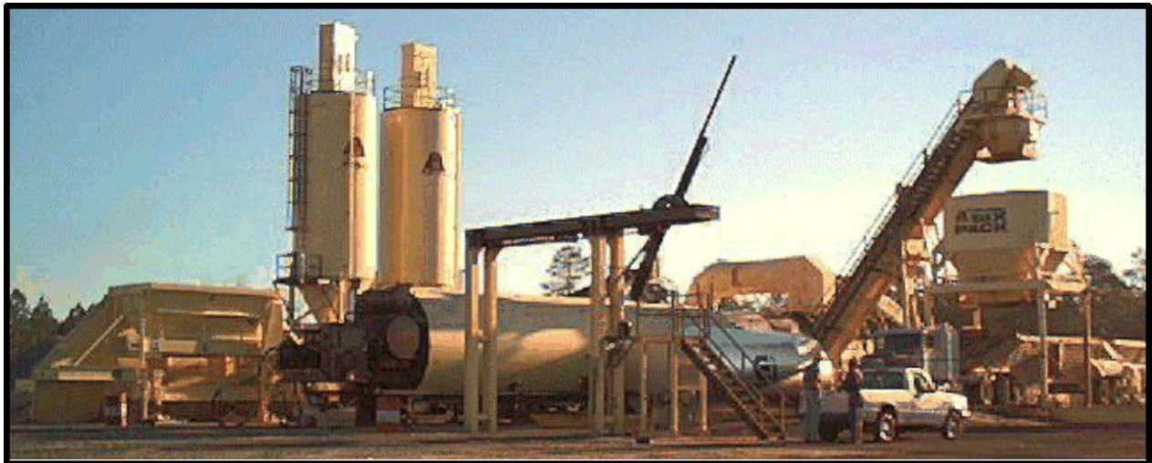
Figure 2 – Onsite Plant at Track (Robotic Sampling Device in Foreground)
