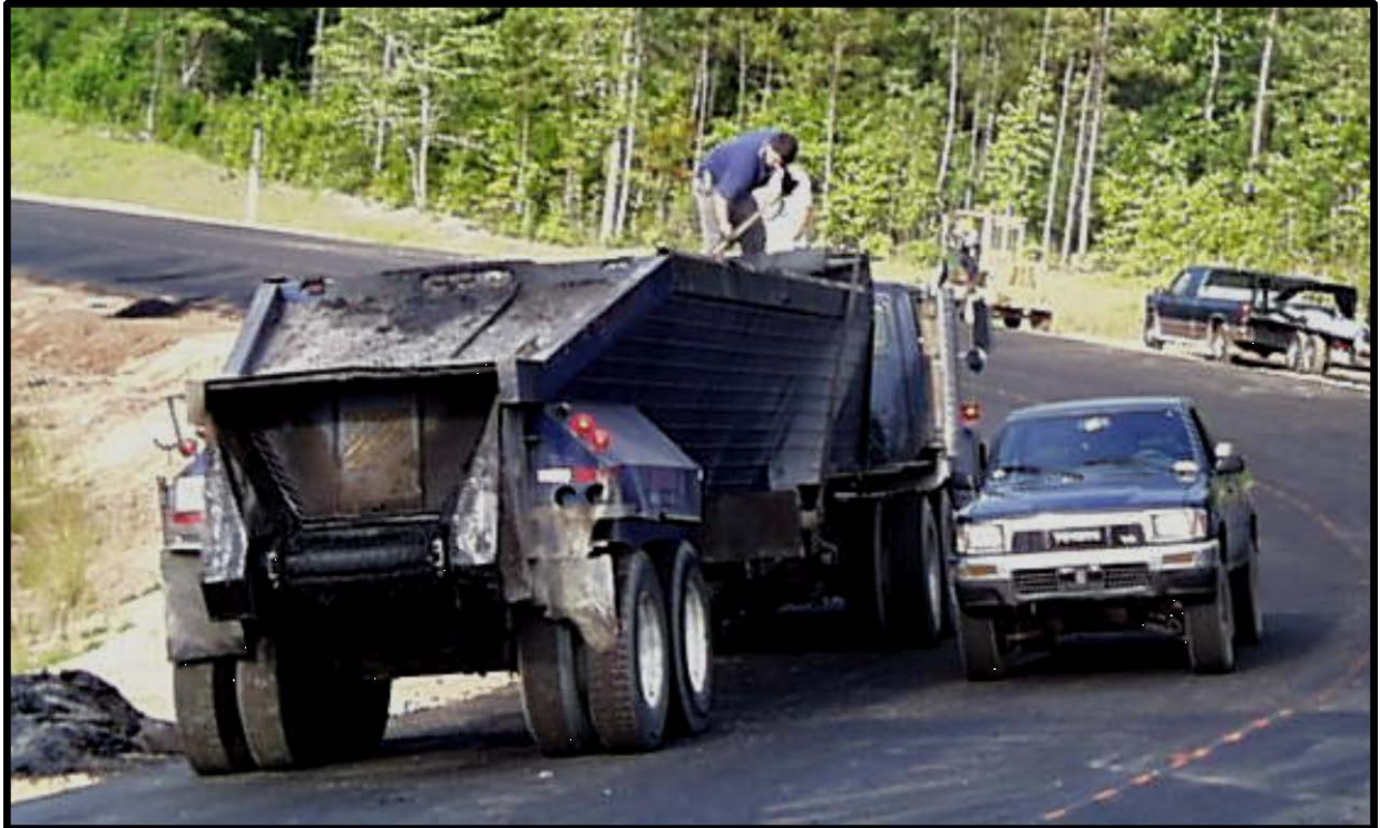
Figure 6 – Removing a Shovel Sample from Flow-Boy Truck on Roadway
